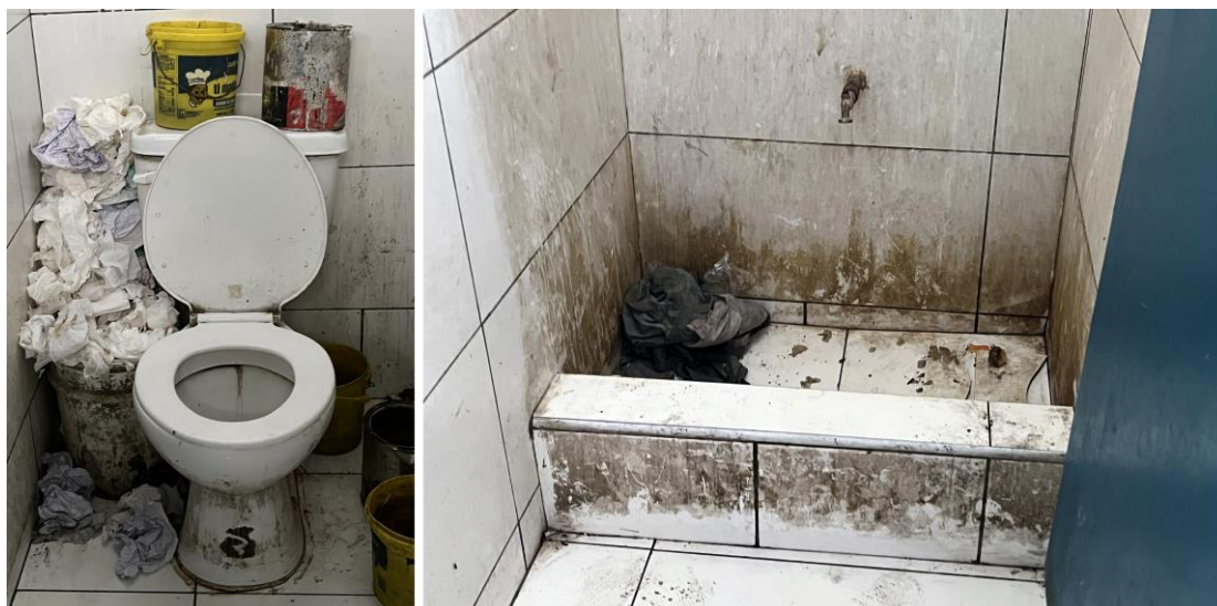
During their September 2024 visit, Amnesty International's researchers observed how sanitation facilities in displacement sites were not accessible to persons with disabilities. © Amnesty International
