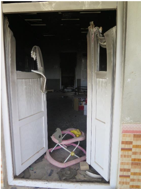
Looted and burned down house in Jiri © Amnesty International
